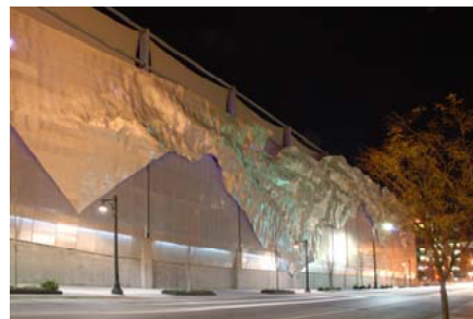
Bartle Hall North Dock
