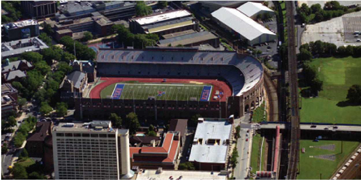
An aerial view of Franklin Field before construction began.
